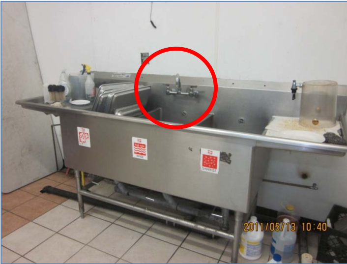
A1a. Three compartment sink: faucet neck does not reach all three compartments.
